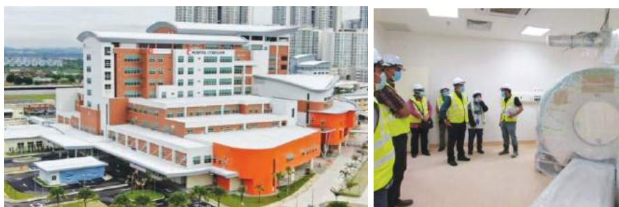
Image 6.40 Main Block of Cyberjaya Hospital (9 storeys) and CT Scanner Machine
