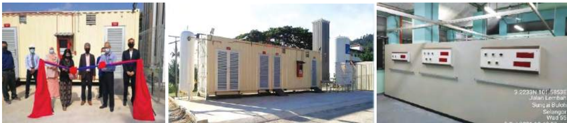
Image 6.17 Construction of Medical Gas System Facilities at PKKN, Hospital Sungai Buloh
